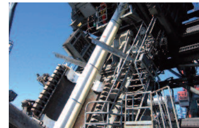
Pipe & CPS Banding
